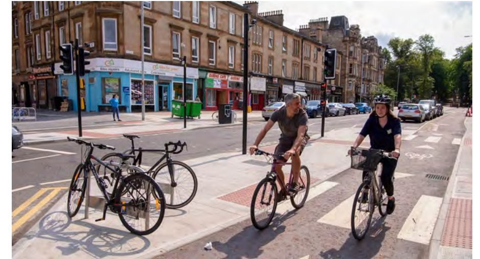
Protected cycle track, catering for side-by-side cycling
